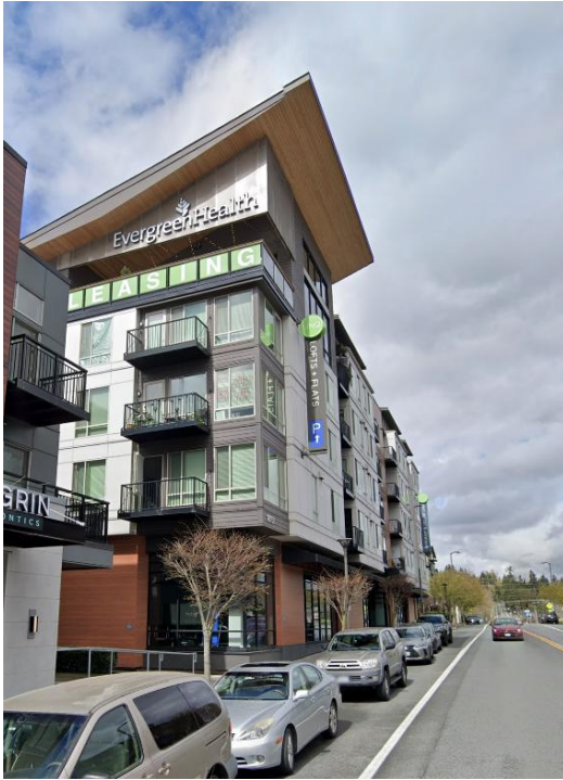
Figure 18. Linq Apartments on 68 th Avenue NE
