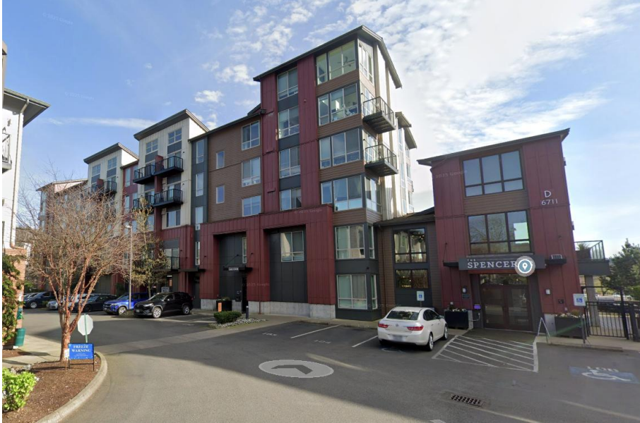
Figure 17. North façade of Building D in Spencer 68
