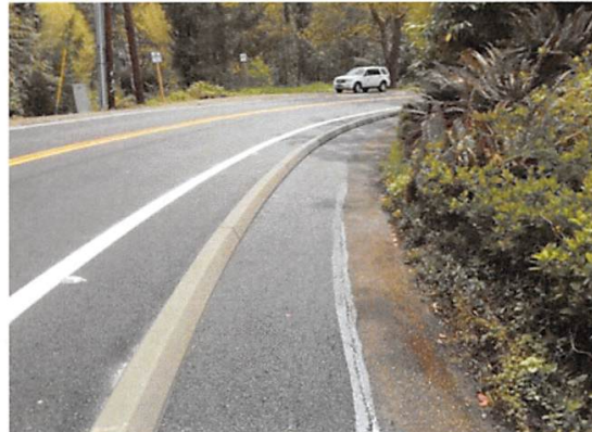
Arrowhead Drive – After curve changes (looking east)
