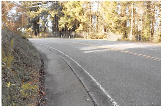
Arrowhead Drive – Before curve changes (looking north)
