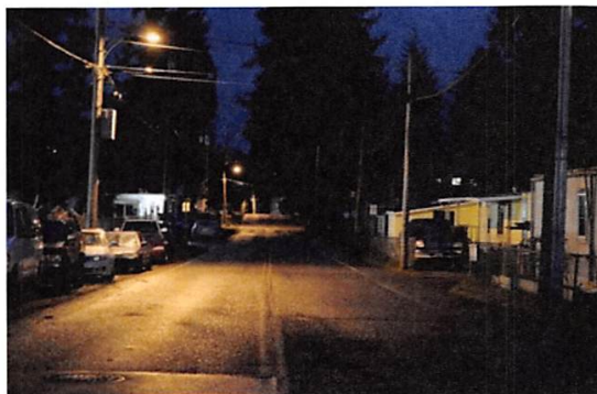
NE 182 nd Street – before lighting upgrades
