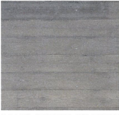
BOARD FORMED CONCRETE
