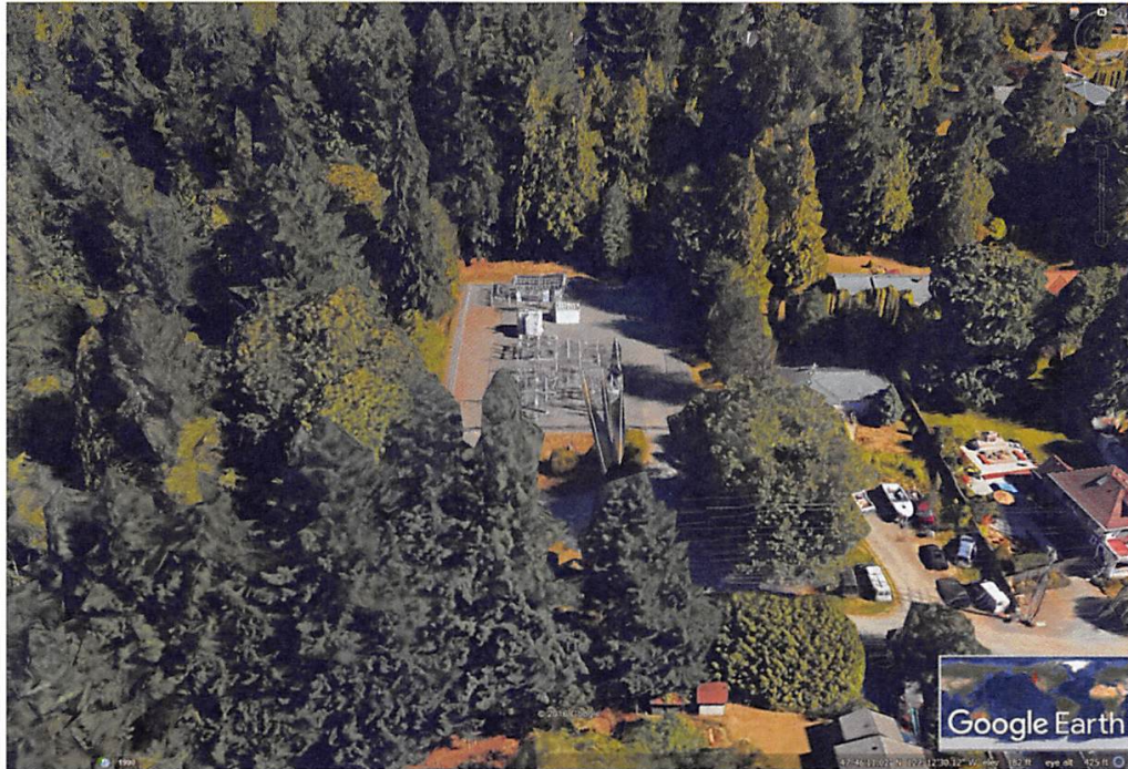
Figure 7. The North Bothell substation.
