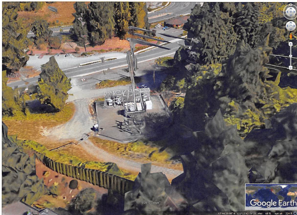
Figure 6. Wayne substation along 96 th avenue NE close to the Red Brick Road intersection
