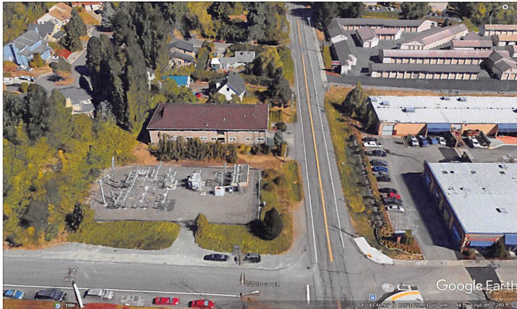
Figure 3. Google Earth view of the Kenmore substation
