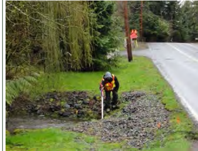
Culvert at NE 192 nd Street (downstream side)
