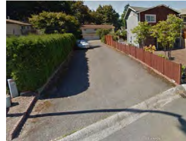
71 st Place NE – location of underground detention tank
