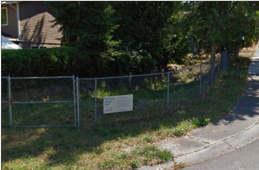
Figure 9: Bixby Knoll Stormwater Pond 2
