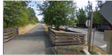
Diversion structure at Burke-Gilman Trail at NE 175 th Street, looking east
