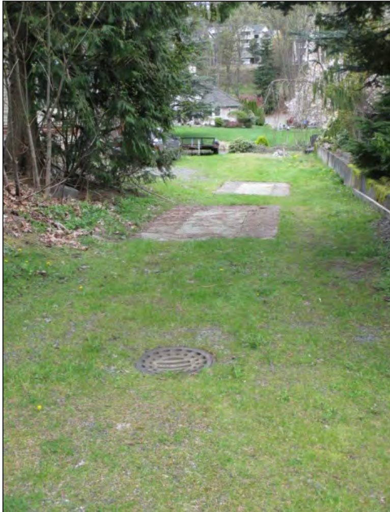
Figure 6: Sammamish River Vaults
