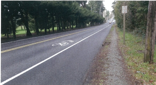
Existing Conditions on Juanita Drive
