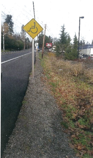
Location of Cantilevered Sidewalk
