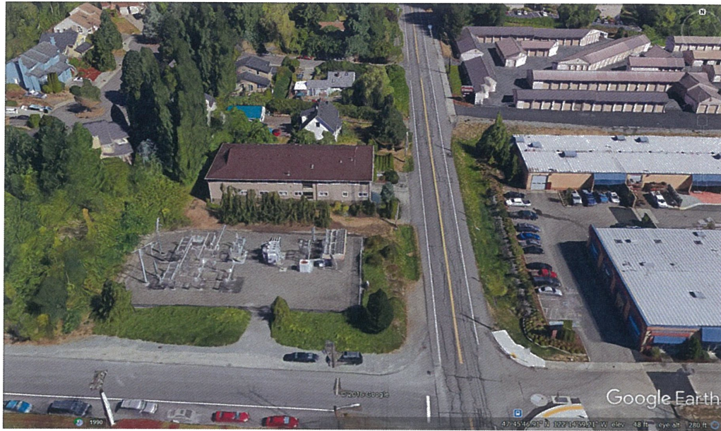
Figure 3. Google Earth view of the Kenmore substation
