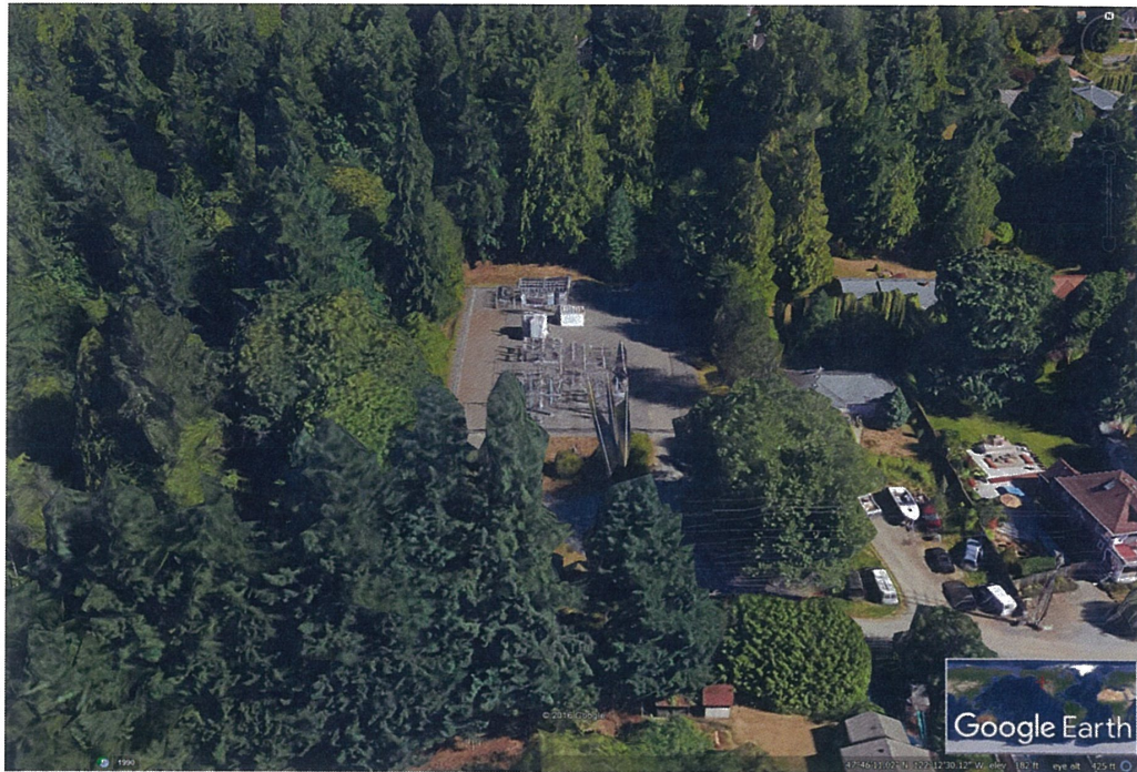
Figure 7. The North Bothell substation.
