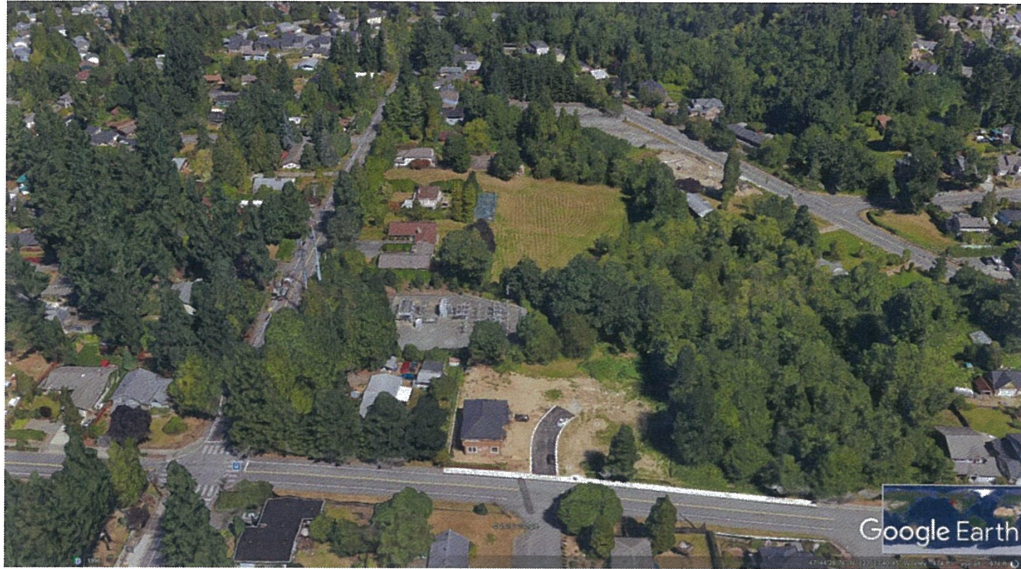
Figure 5. Inglewood substation at NE 155 th street and 84 th avenue NE
