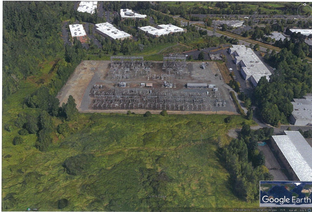
Figure 8. Sammamish bulk power substation along Willows Rd in Redmond
