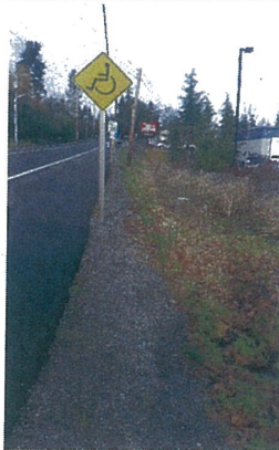
Location of Cantilevered Sidewalk
