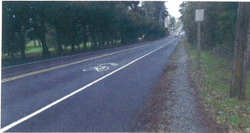
Existing Conditions on Juanita Drive
