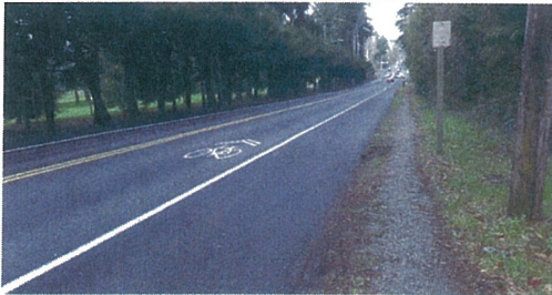
Existing Conditions on Juanita Drive
