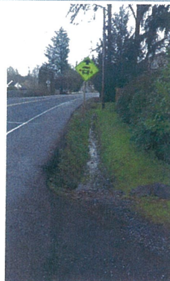
West side of 68 th Ave NE
