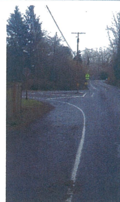
The project will meet the Safe Routes to School project
