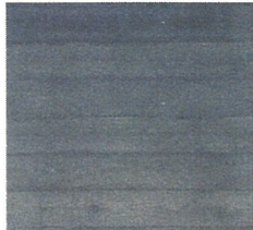
BOARD FORMED CONCRETE
