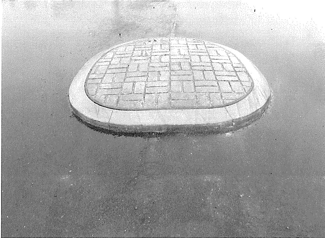
Figure 9 – Sample Stamped Concrete Island – 67 th Avenue NE and NE 181 st Street
