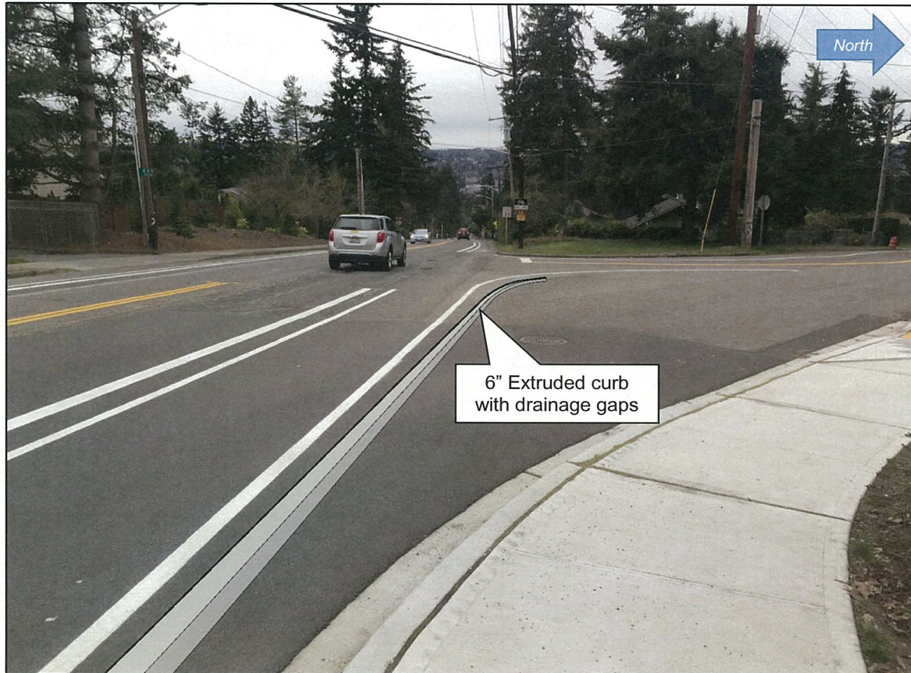
Figure 1 – Extruded Curb Treatment
