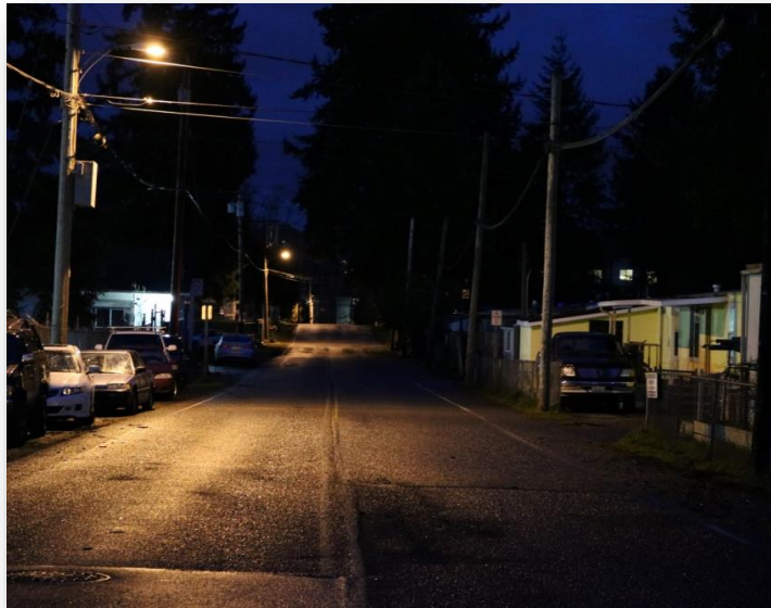
NE 182 nd Street Before
