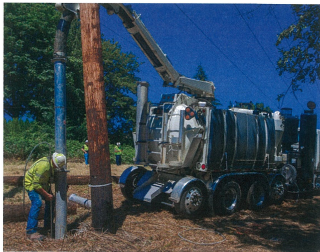
In 2016, we coordinated with Olympic Pipe Line Company on the work plan and safe construction practices to replace two poles in Newcastle.
