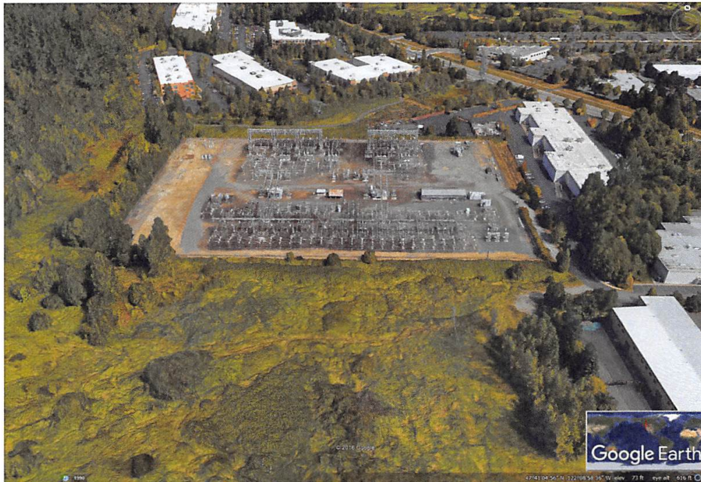
Figure 8. Sammamish bulk power substation along Willows Rd in Redmond
