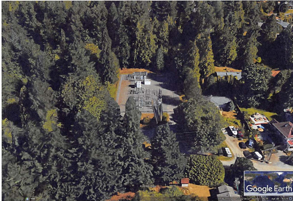
Figure 7. The North Bothell substation.
