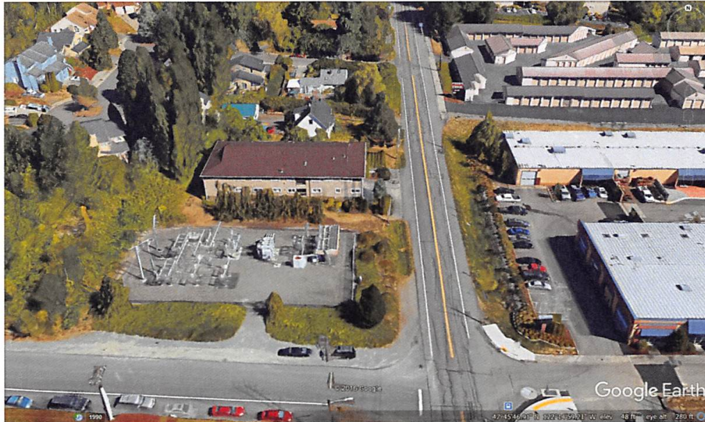
Figure 3. Google Earth view of the Kenmore substation
