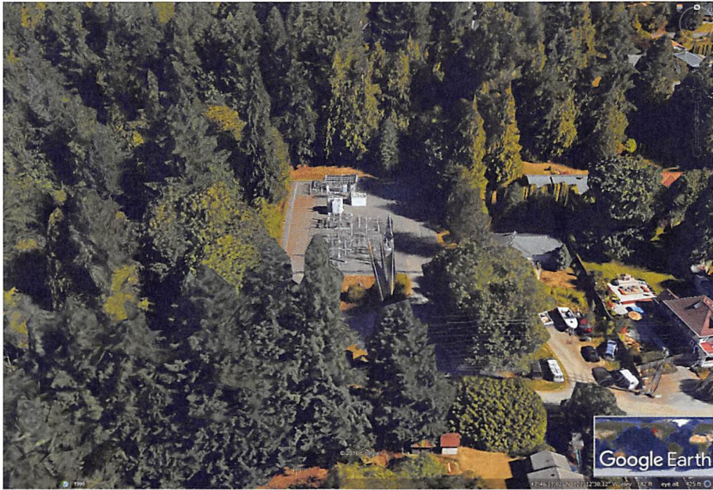
Figure 7. The North Bothell substation.
