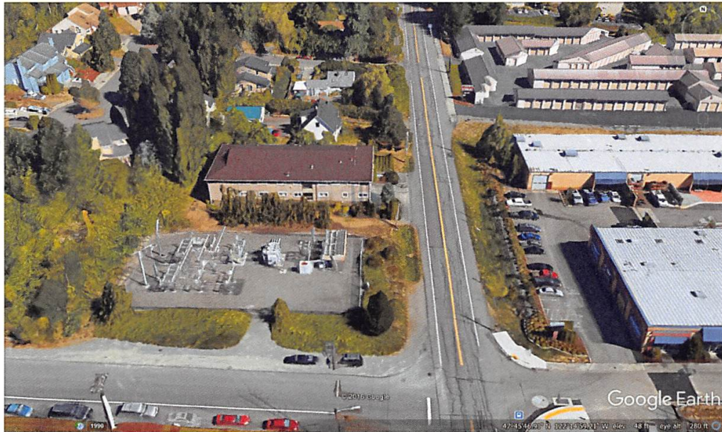
Figure 3. Google Earth view of the Kenmore substation
