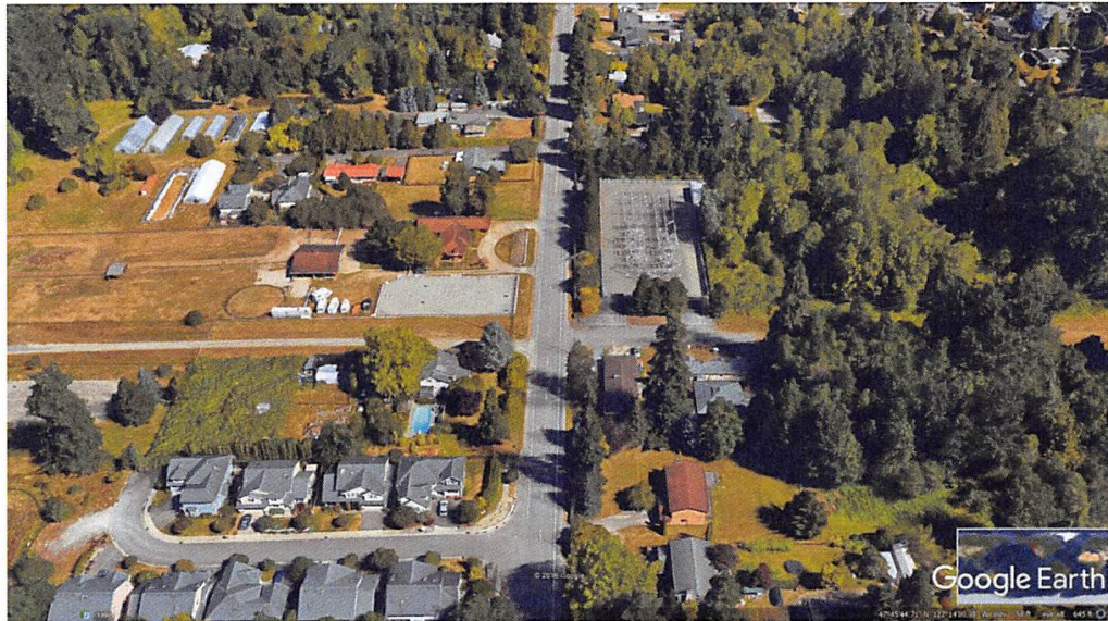
Figure 4. Moorlands switching station at NE 185 street and 80 th avenue NE
