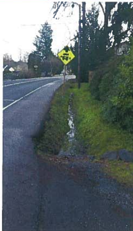
West side of 68 th Ave NE
