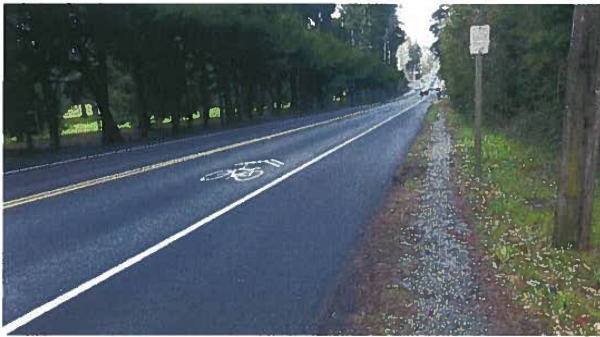
Existing conditions on Juanita Drive
