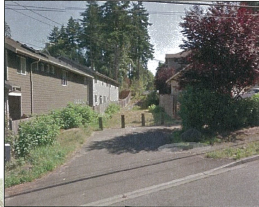
Cort Ridge Detention Tank and Bioswale
