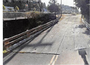
Figure A: Existing Bridge
