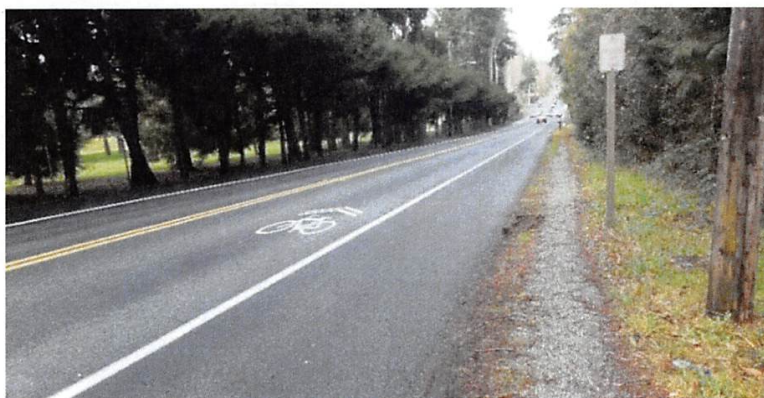
Existing Conditions on Juanita Drive
