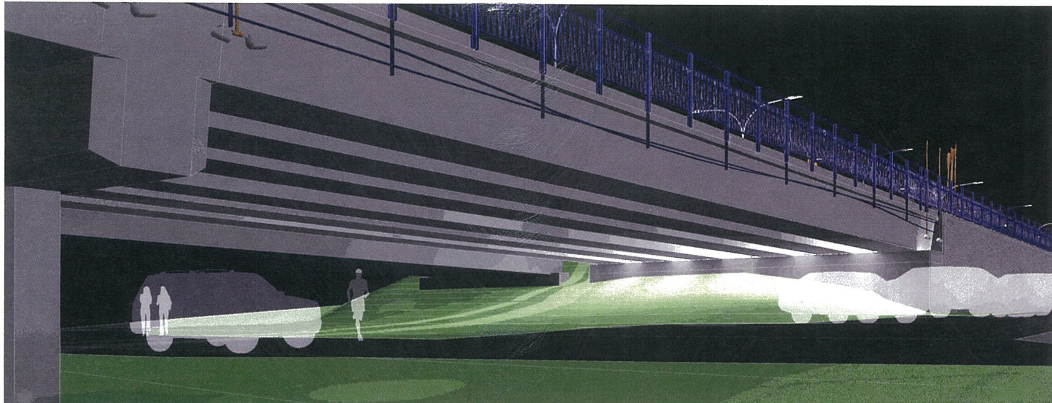
VIEW LOOKING SOUTHEAST TOWARD SOUTHERN BRIDGE ABUTMENT. INDIRECT LIGHTING ELEMENTS BETWEEN TUB GIRDERS ILLUMINATE BRIDGE UNDERPASS
