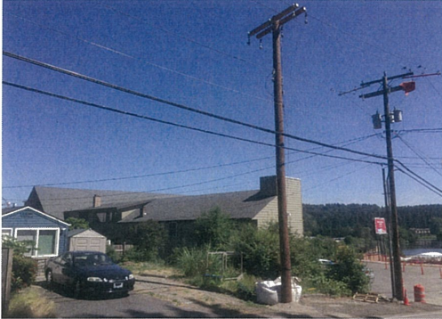
Picture #1 - Current Pole Configuration (Looking East)
