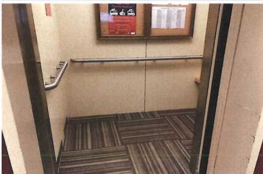
#29 ELEVATOR CAB FINISHES
