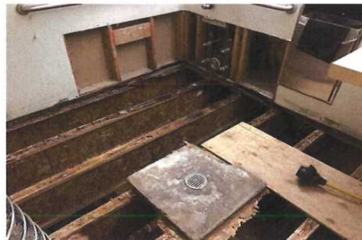
#6 WOOD SUBFLOORING - FRONT RESTROOM REMEDIATION
