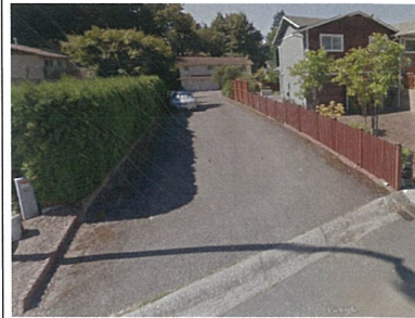
Detention tank underneath 71 st Pl. NE.
