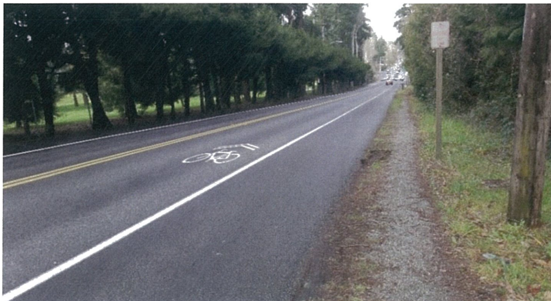
Existing Conditions on Juanita Drive
