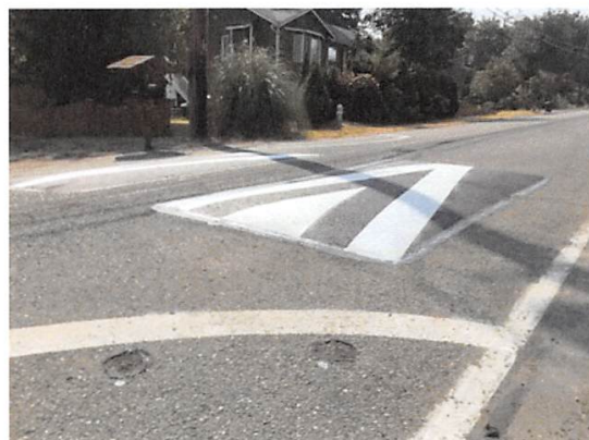
75 th Avenue NE – speed cushions (west shoulder, looking north near NE 153 rd Place)
