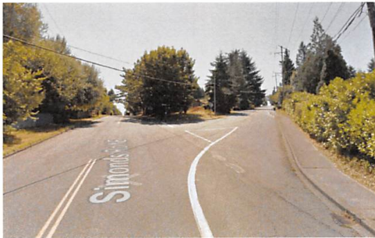
84 th Avenue and Simonds before modification
