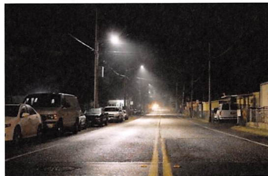
NE 182 nd Street – after lighting upgrades
