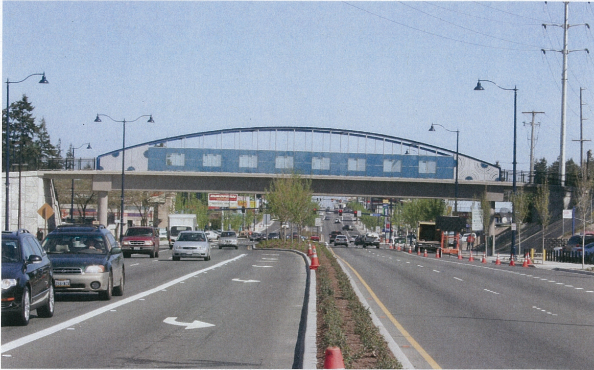
Figure 1. Aurora Avenue N Bridge, Shoreline
