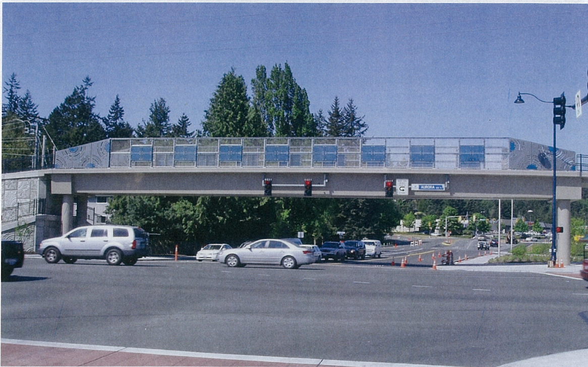
Figure 2. N 155th St Bridge, Shoreline
