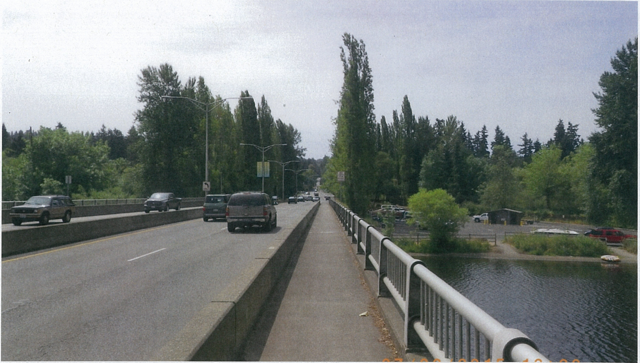
Figure 7. Pedestrian View Looking South
