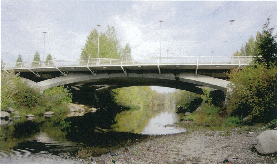
Figure 3. NE 190th St Bridge, Redmond
