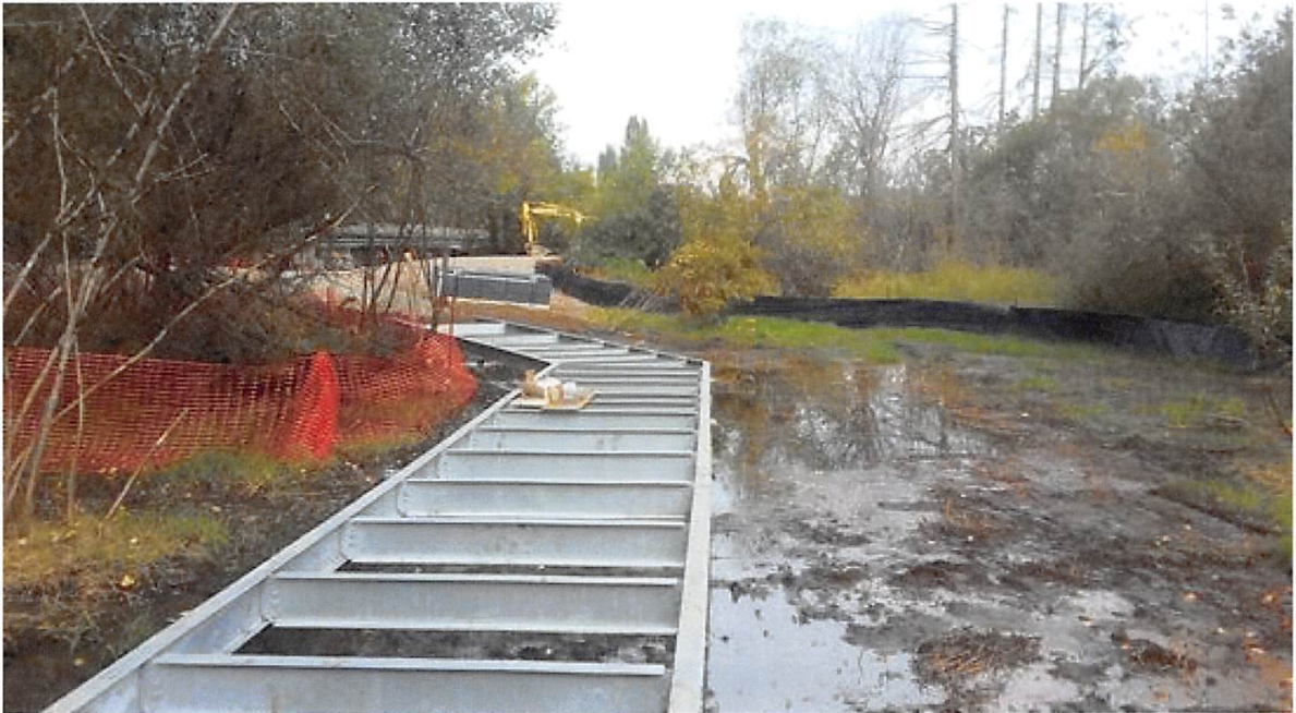
Waterwalk under construction in early October.
