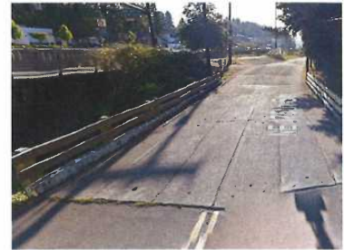
Figure A: Existing Bridge
