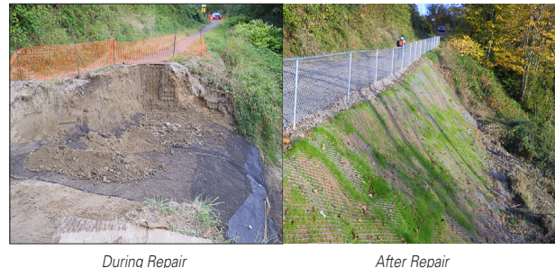
Emergency Evacuation Trail, Sultan, Washington
