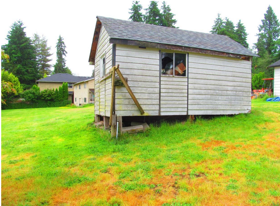
Large storage shed exterior, facing east
