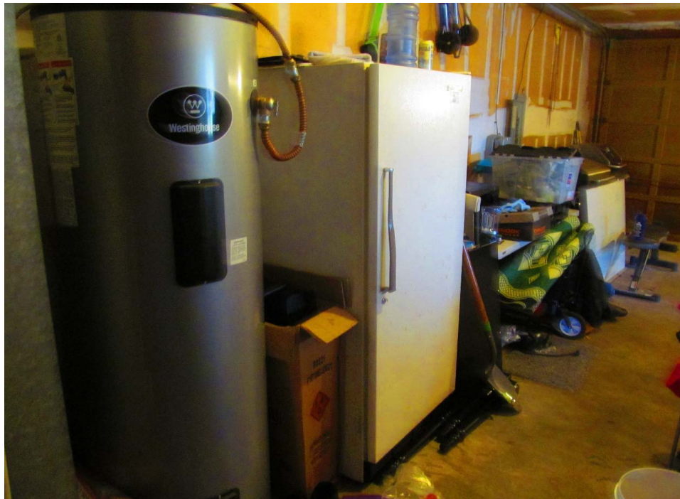
Single-family residence interior, garage
