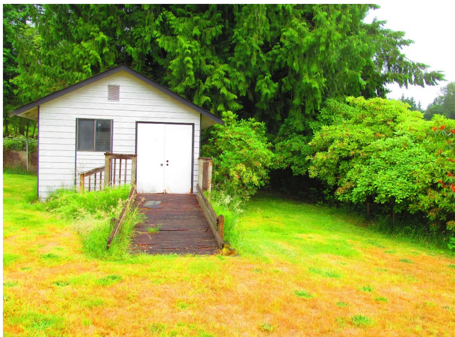
Property exterior with view of tool shed exterior, facing west
