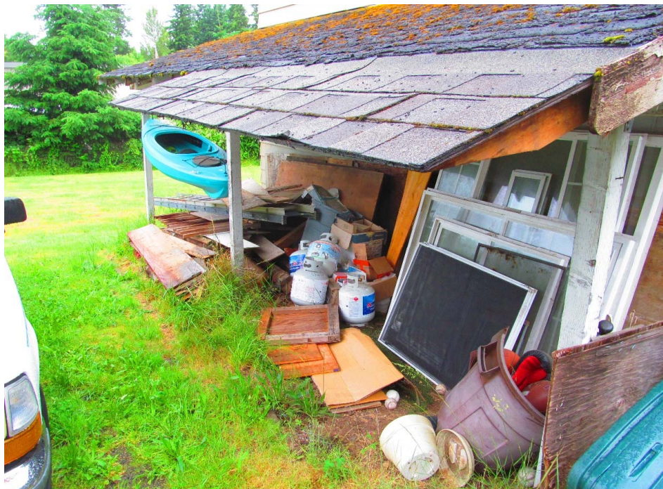
Exterior storage outside of workshop/apartment
