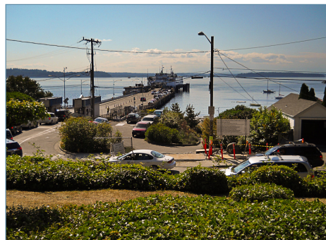
Barton Pump Station, Seattle, Washington
