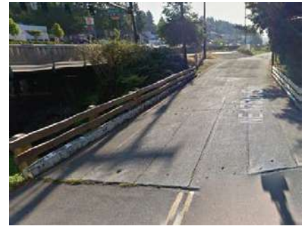
Figure A: Existing Bridge
