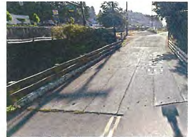
Figure A: Existing Bridge
