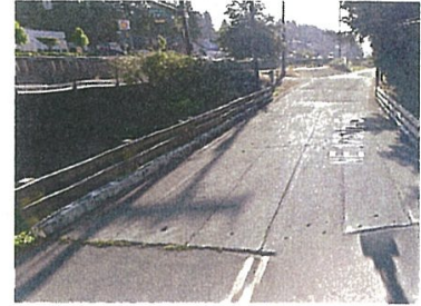
Figure A: Existing Bridge
