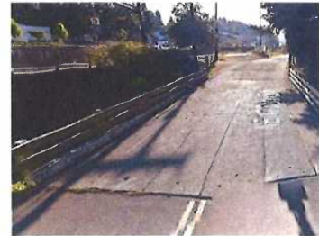
Figure A: Existing Bridge
