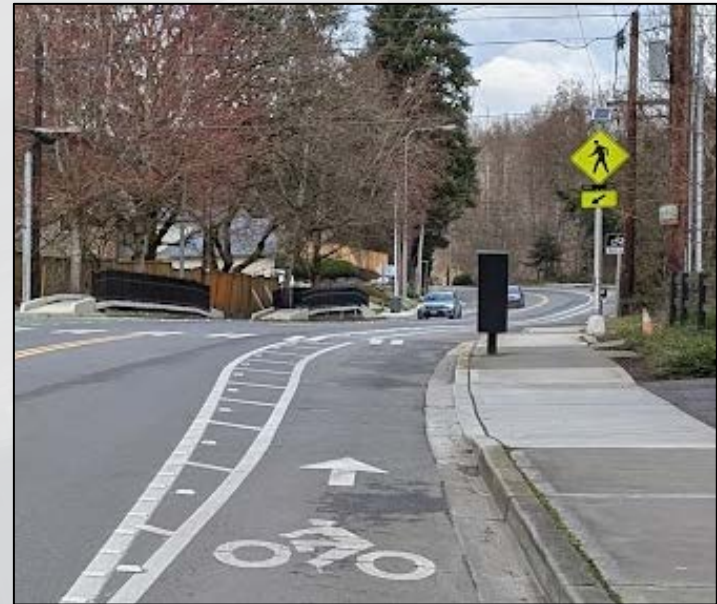
Buffered Bike Lane on 73 rd Ave
