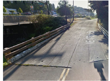
Figure A: Existing Bridge
