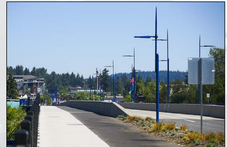
West Sammamish Bridge Path
