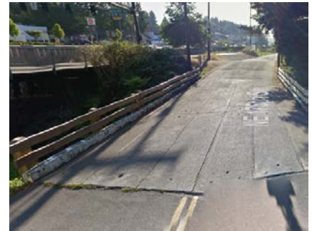
Figure A: Existing Bridge
