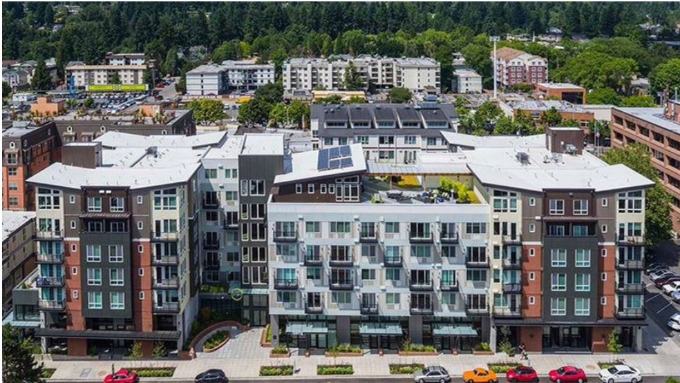
7 story, Origin Apartments, Lake City
