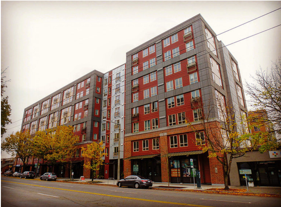
8 story mixed use building, Ballard (Photo credit: Dan Bertolet, Sightline)
