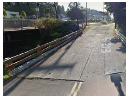
Figure A: Existing Bridge
