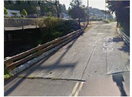
Figure A: Existing Bridge
