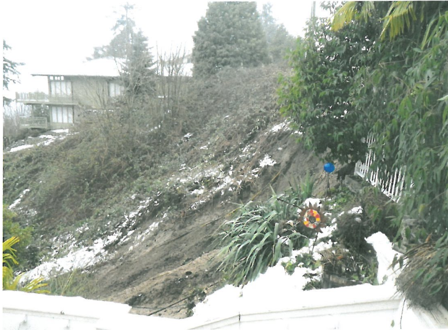
Photo #3: Slide area from 15219 NE 61 st Place NE (facing north)
