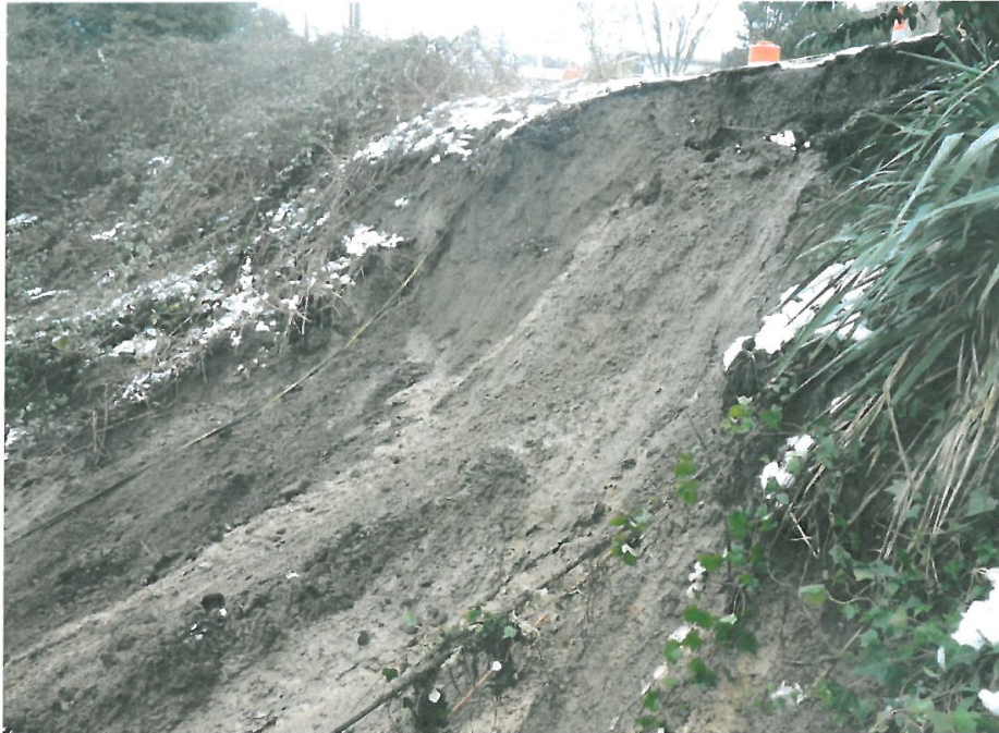
Photo #5: Slide area from 15219 NE 61 st Place NE (facing north-east)
