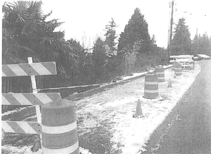
Photo #1: 61 st Place NE above slide area (facing north)
