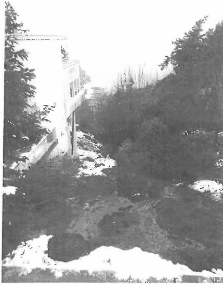
Photo #8: Slide area from NE 61 st Place NE (facing west)
