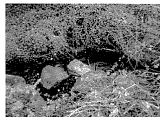
Rocks from wall which fell into the stream.
