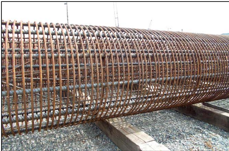
Rebar cages built in Kenmore for Pier 36 columns.
