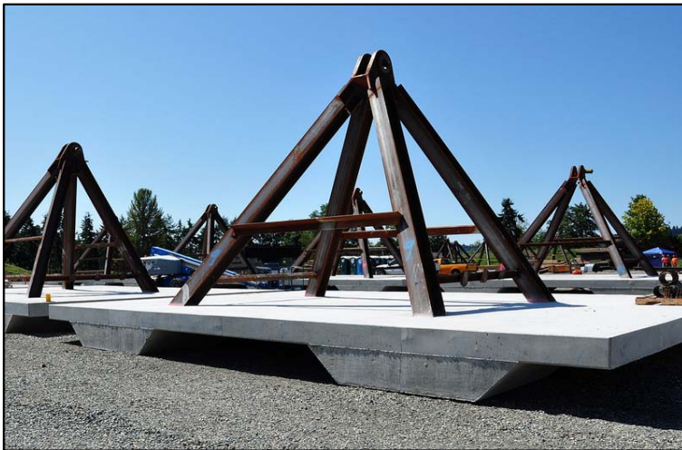
Completed fluke anchors await transport to the floating bridge site in August 2012.
