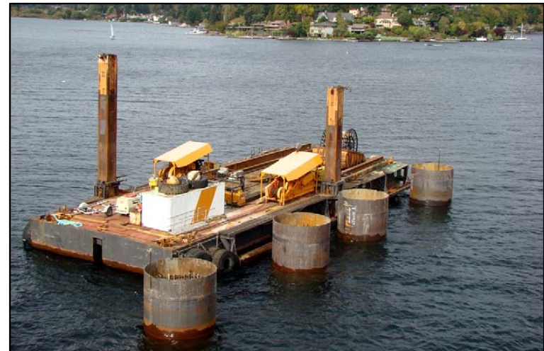
Shafts for the support columns of Pier 36 near Madison Park.
