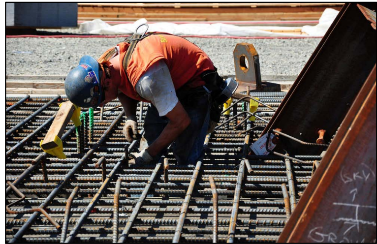
A worker ties rebar for the base of a fluke anchor in August 2012.
