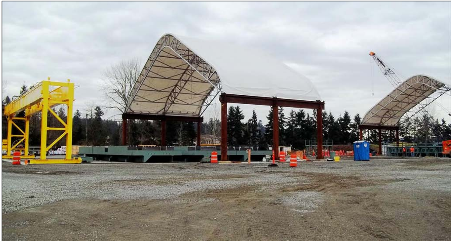
The roadway deck panel casting area in February 2013. Casting of the deck panels is expected to begin winter 2013/2014.
