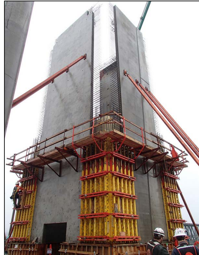
Once complete, the box column panels were installed in their final locations on Pontoon W near Medina in January 2013.
