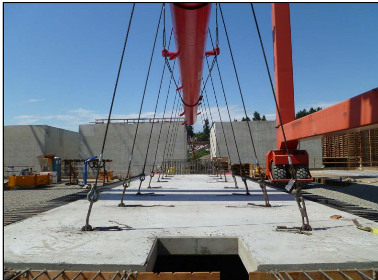
In Kenmore, a crane carrier hoists a completed box column wall panel in August 2012. The second set of gravity anchors can be seen in the background.
