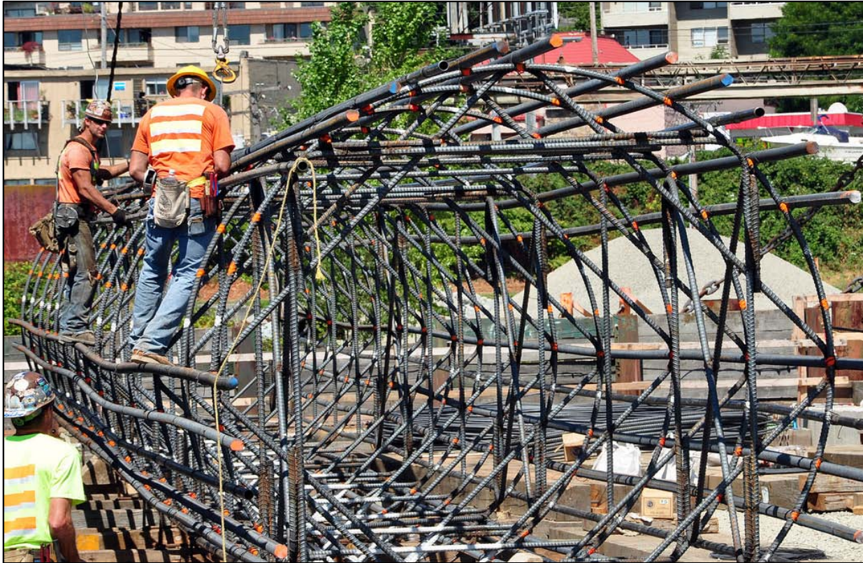
Workers construct the rebar cage for a cast-in-place shaft anchor at the Kenmore site in August 2012.
