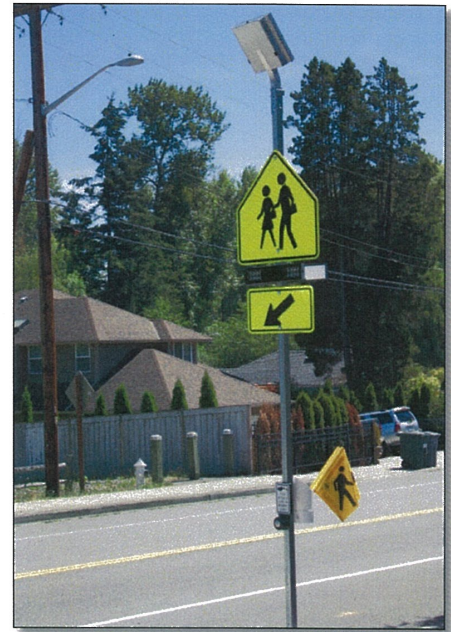
Rectangular Rapid Flash Beacon at 73rd Ave NE near Kenmore Elementary
