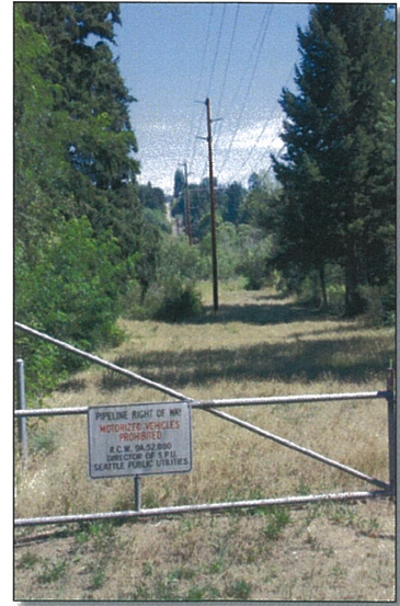
Portion of Tolt Pipeline Trail, Looking East at 73 rd Ave NE
