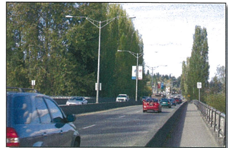
North Side of Sammamish River Bridge
