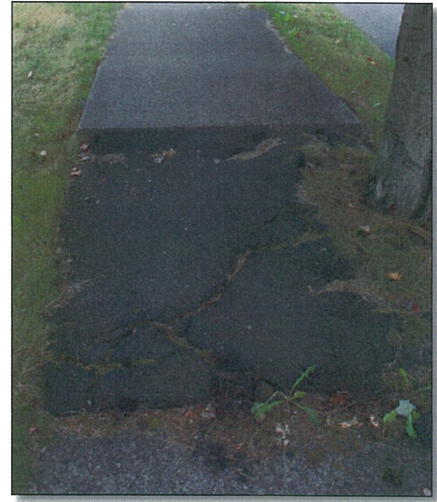
Sidewalk on 61 st Ave NE
