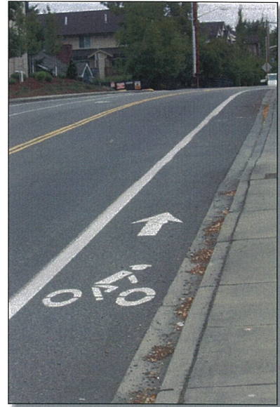
Example of a bike lane on NE 80 th Ave
