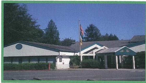
Figure 3.15 Photo: Kenmore Elementary School
