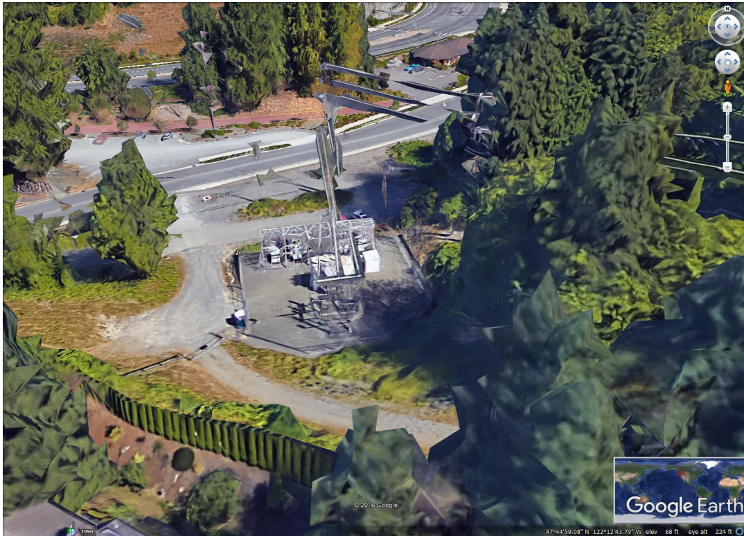
Figure 6. Wayne substation along 96 th avenue NE close to the Red Brick Road intersection
