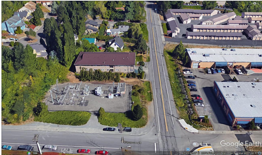
Figure 3. Google Earth view of the Kenmore substation
