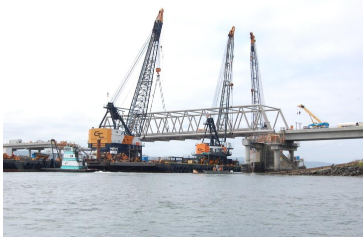
EXHIBIT 1-17. THREE LARGE CRANES LIFTING A TRUSS INTO PLACE FROM A BARGE
