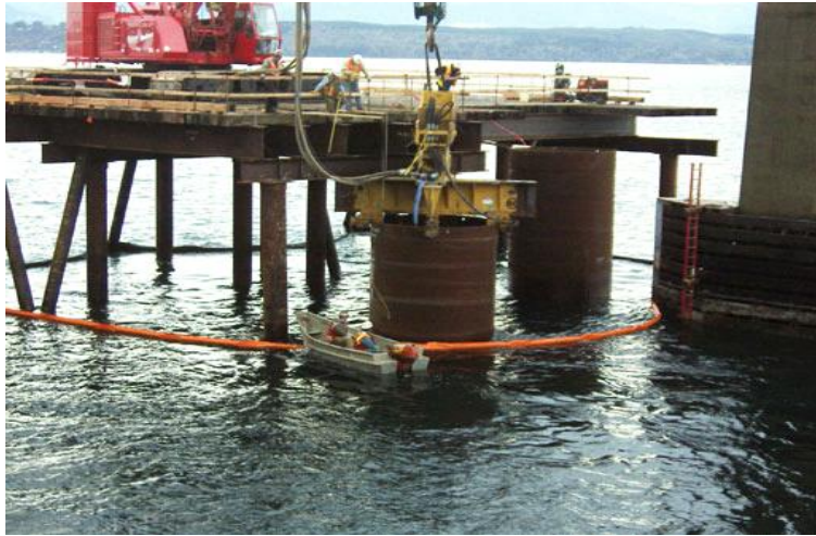
EXHIBIT 1-7. DRILLED SHAFT CASING INSTALLATION WITH A VIBRATORY HAMMER
