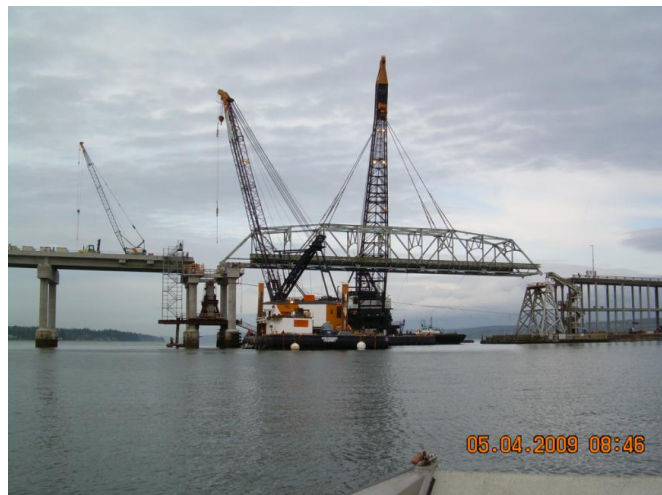
EXHIBIT 1-20. REMOVAL OF THE HOOD CANAL BRIDGE TRANSITION TRUSS
