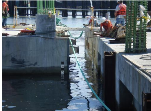
EXHIBIT 1-16. ROPES, WINCHES, AND ASSOCIATED TACKLE BEING USED TO ALIGN PONTOONS AND BRING THEM TOGETHER (FROM THE HOOD CANAL FLOATING BRIDGE PROJECT)
