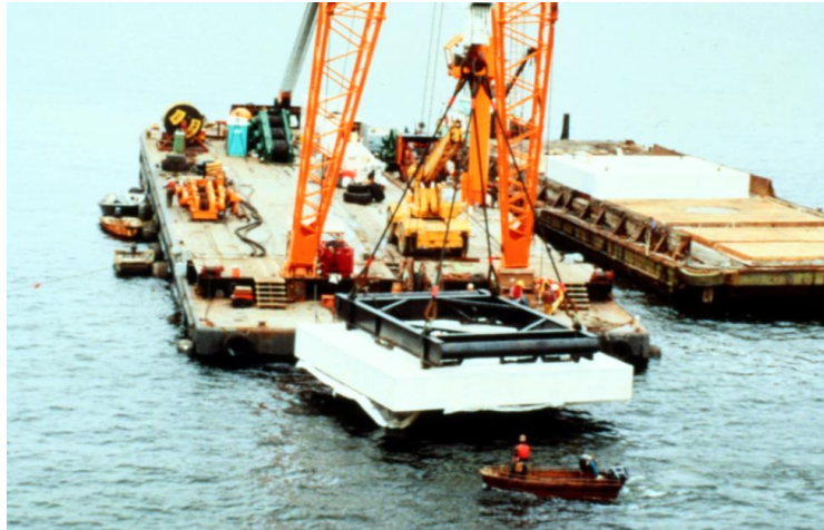
EXHIBIT 1-13. GRAVITY ANCHOR SEGMENT INSTALLATION FOR THE LACEY V. MURROW PROJECT
