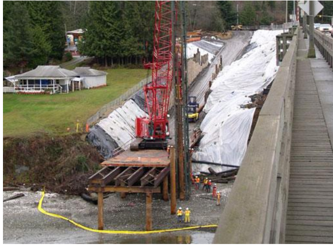
EXHIBIT 1-4. WORK BRIDGES ON PILE-DRIVING CRANES
