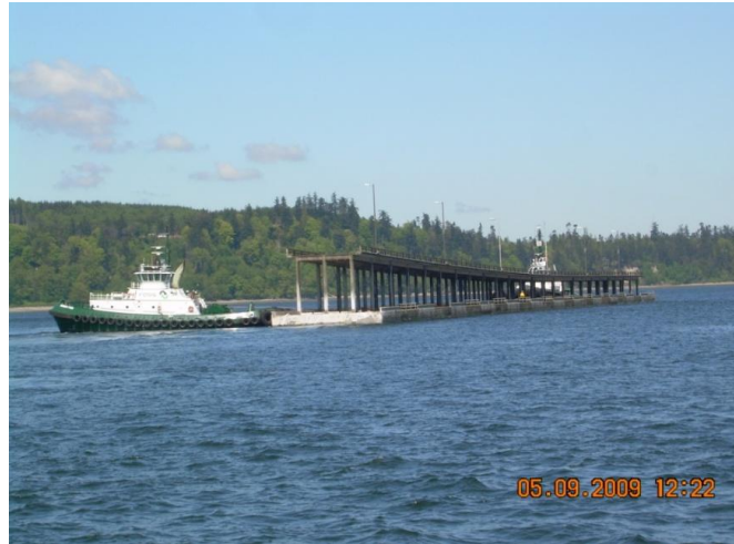
EXHIBIT 1-22. PONTON UNDER TOW, WITH THE ELEVATED SUPERSTRUCTURE INTACT
