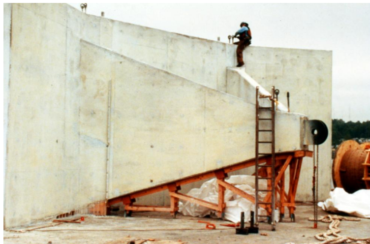
EXHIBIT 1-12. FLUKE ANCHORS CONSTRUCTED FOR THE LACEY V. MURROW PROJECT
