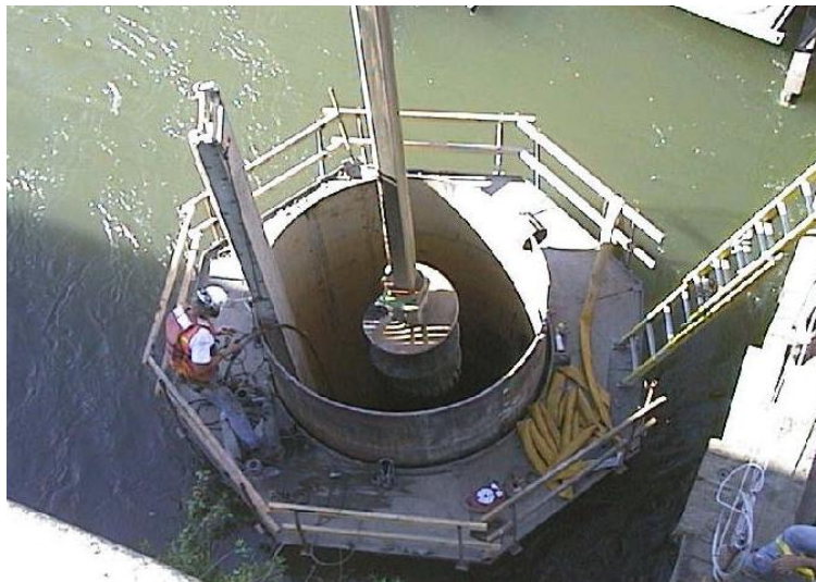
EXHIBIT 1-8. AUGER USED FOR EXCAVATING SOILS INSIDE THE DRILLED SHAFT CASING
