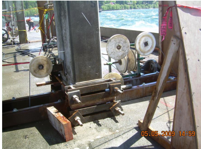
EXHIBIT 1-18. CUT-WATER CONTAINMENT SYSTEM FOR CUTTING A PONTOON JOINT
