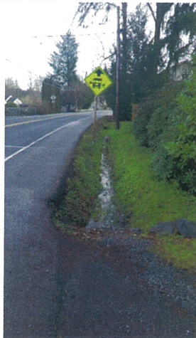
West side of 68 th Ave NE
