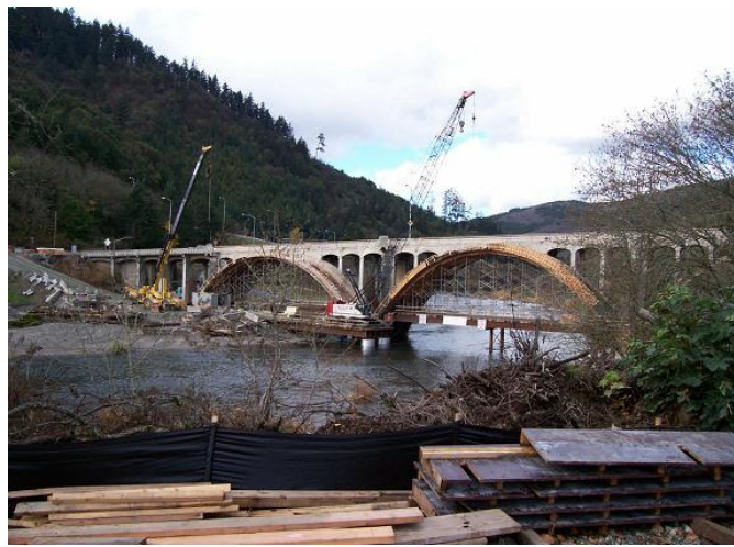
EXHIBIT 1-5. FALSEWORK, TEMPORARY STRUCTURE TO SUPPORT PERMANENT BRIDGE STRUCTURES
