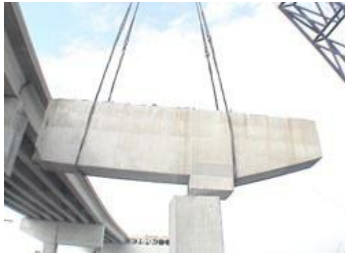
EXHIBIT 1-19. BRIDGE CROSS BEAM SECTION BEING LIFTED BY CRANE AFTER SAW CUTTING THROUGH COLUMN AND BEAM
