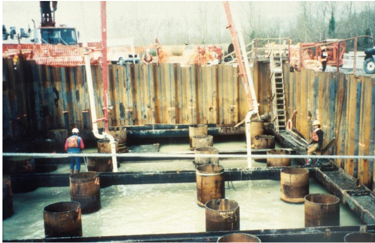
EXHIBIT 1-10. CONCRETE PUMP TRUCKS PLACING UNDERWATER CONCRETE FOR A SEAL INSIDE A COFFERDAM
