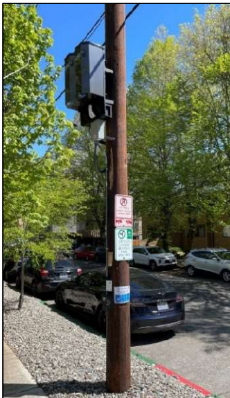
Examples of pole charger installations
