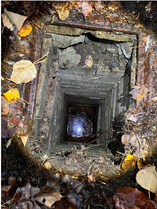
Preexisting Catch Basin
