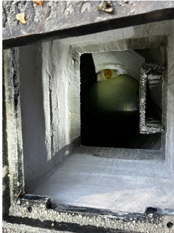
Catch Basin Replaced 2025
