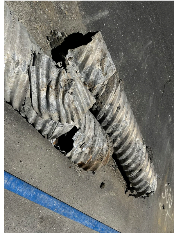
Preexisting Storm Drain
