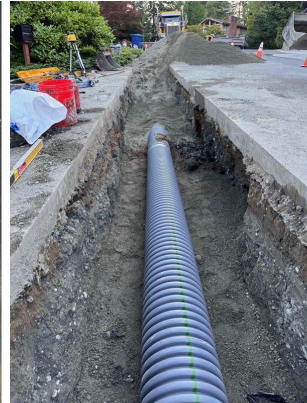
Storm Drain Replaced 2025
