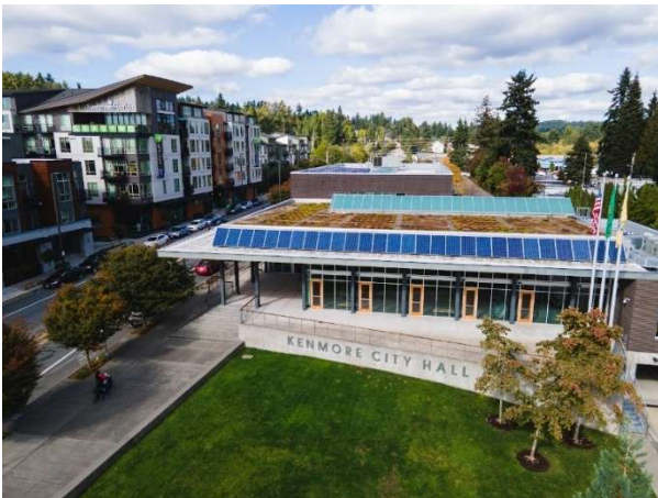
Existing solar on City Hall
