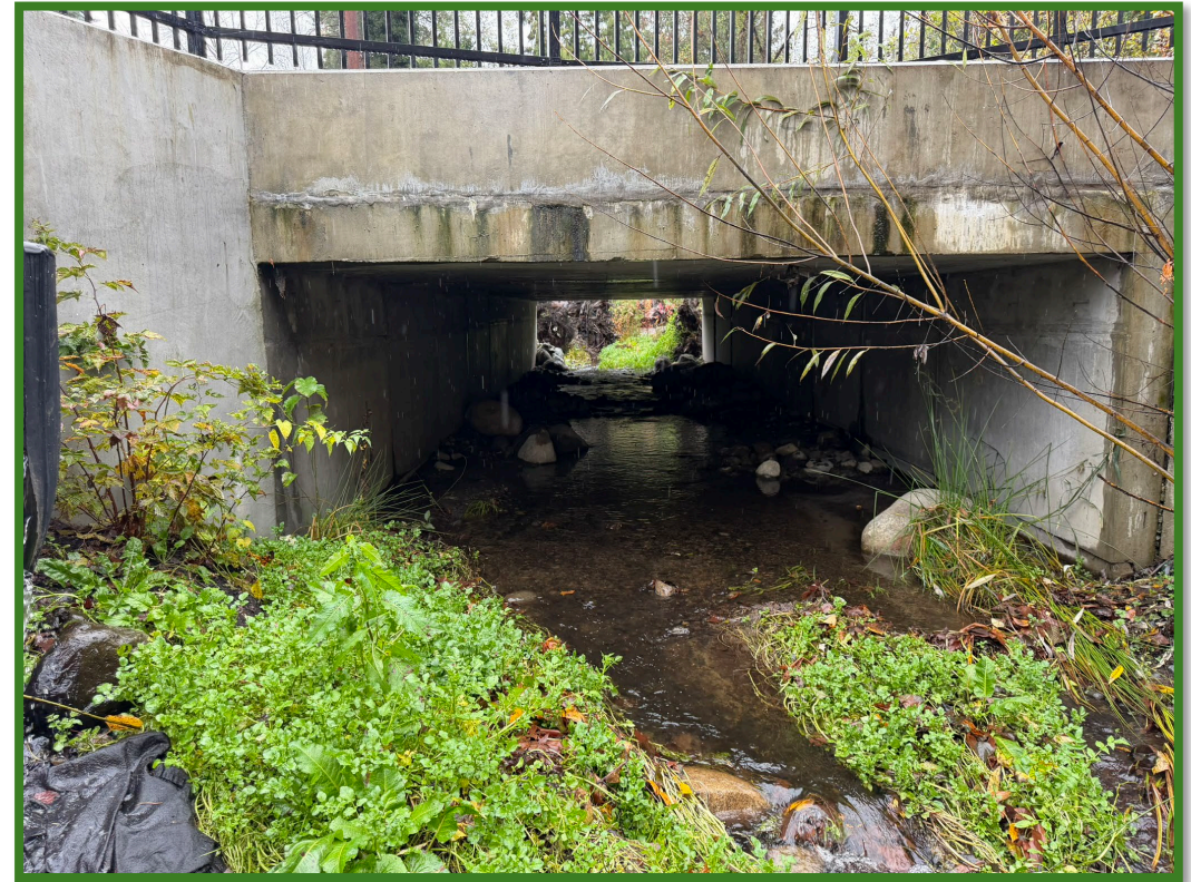
NE 190 th St Culvert Replaced 2023-2024
