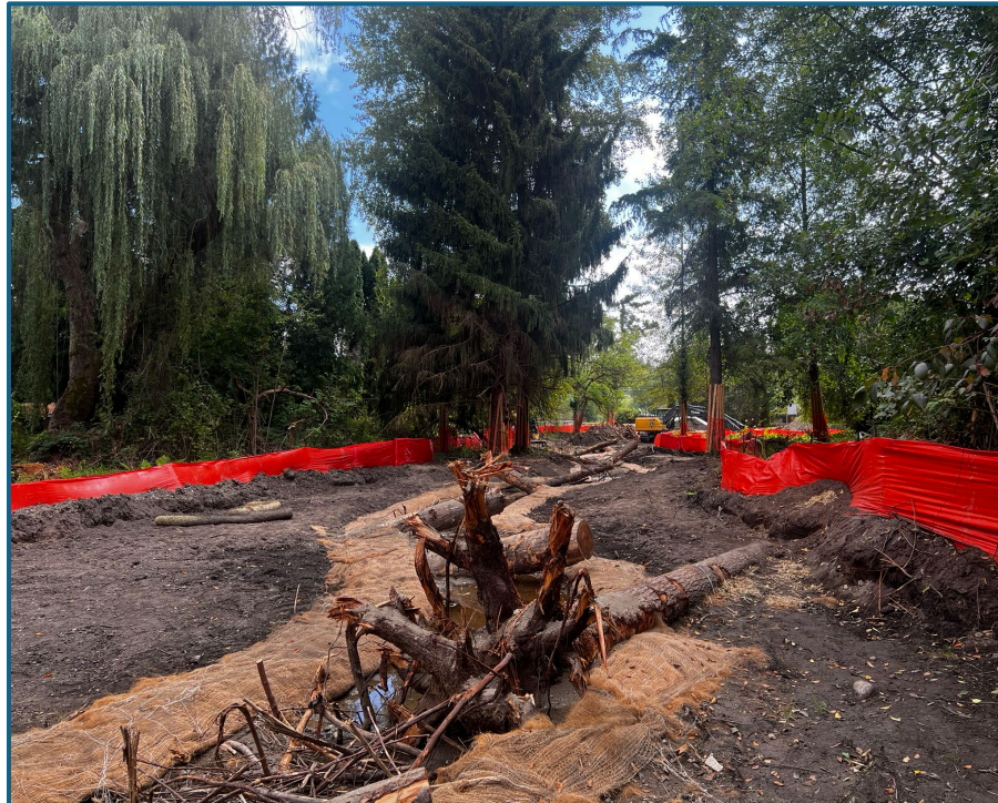
Muck Creek Channel Restoration Construction in Progress
