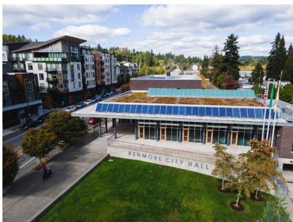
Existing solar on City Hall
