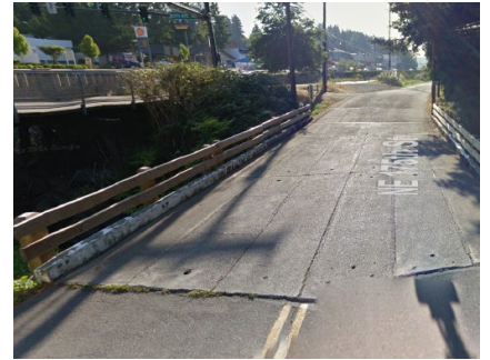
Figure A: Existing Bridge
