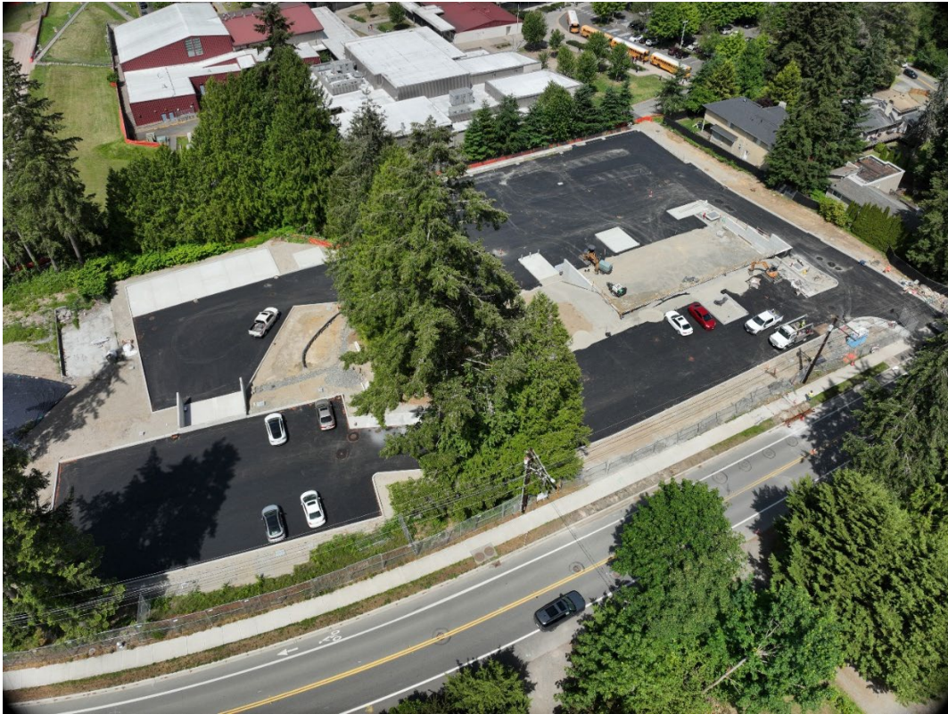
Completion of site work by Contractor #1 at PWOC Site, June 2026
