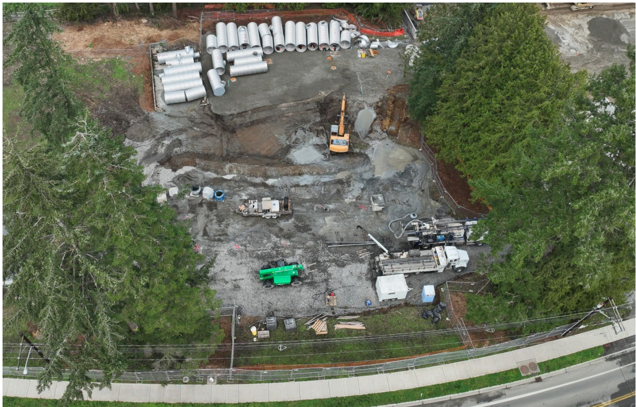
Installation of geothermal wells at PWOC Site, February 2026
